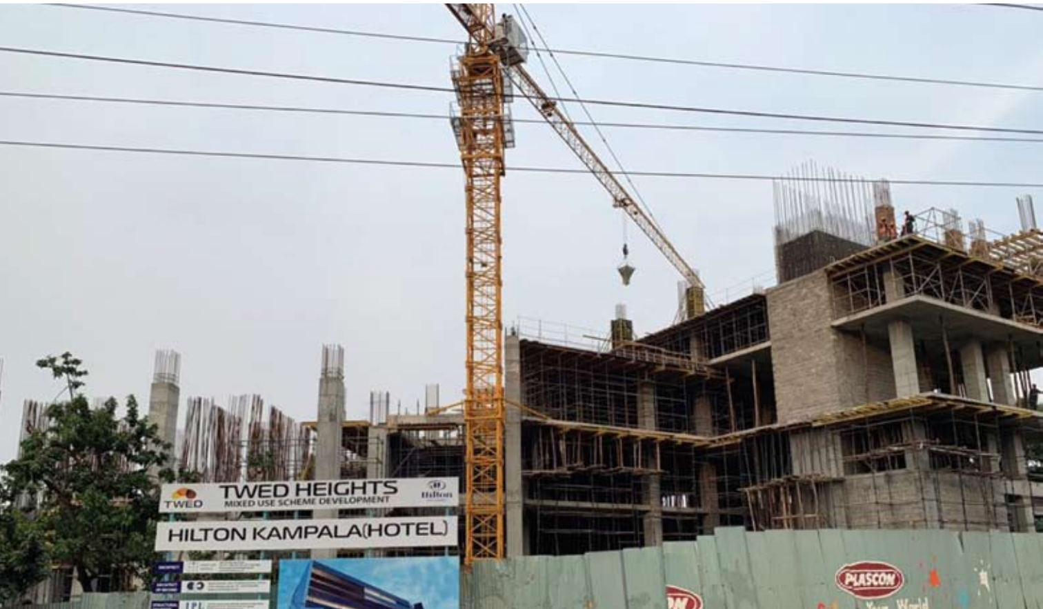
Hilton Hotel under construction by Roko Construction Ltd.
