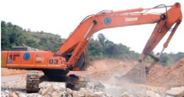
Ongoing works at MKK project by KNWI
